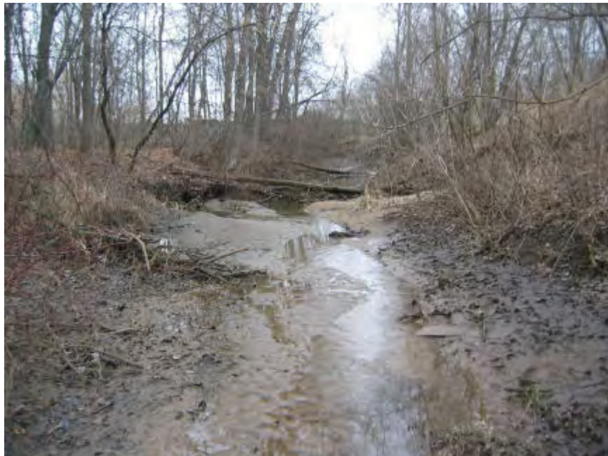
Picture #48 shows the Gilbert and West Town Intercounty Drain in with logjams, debris and heavy sediment build up near Station 133+00 in Section 7, Delhi Township, Ingham County.
