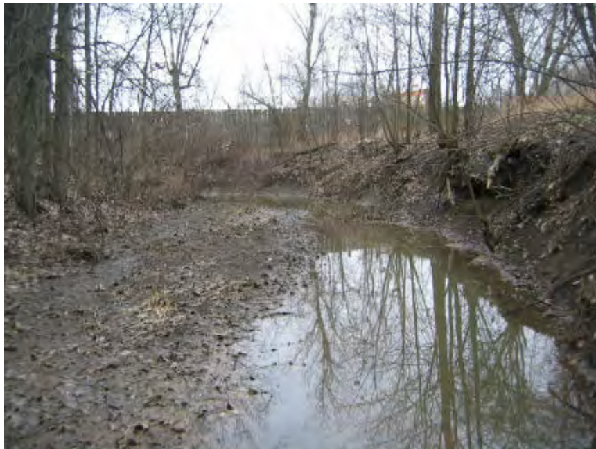
Picture #50 shows the Gilbert and West Town Intercounty Drain with eroded banks and sediment build up near Station 136+50 in Section 7, Delhi Township, Ingham County.
