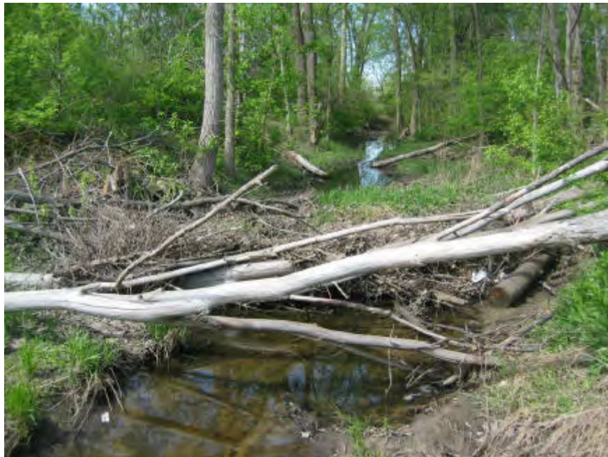
Picture #64 shows the Gilbert and West Town Intercounty Drain with flow obstructions and large fallen trees just north of Bishop Highway near Station 152+00 in Section 7, Delhi Township, Ingham County.
