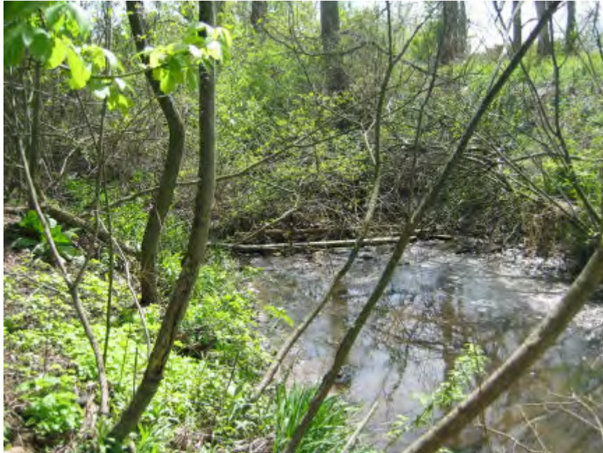
Picture #41 shows the Gilbert and West Town Intercounty Drain in with large fallen trees and logjams near Station 121+00 in Section 18, Delhi Township, Ingham County.
