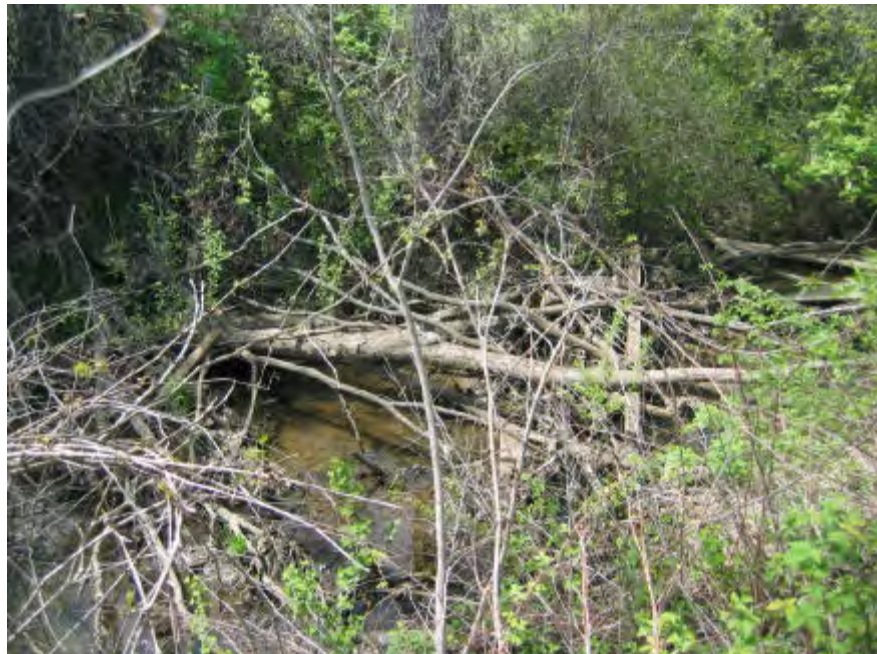
Picture #40 shows the Gilbert and West Town Intercounty Drain in poor condition with large fallen trees and logjams and debris buildup near Station 120+00 in Section 18, Delhi Township, Ingham County.
