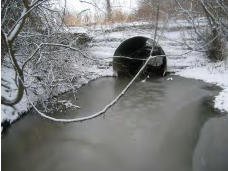
Picture #55 shows a 60" CMP private crossing on the Gilbert and West Town Intercounty Drain near Station 143+50 in Shroyer's Auto Parts in Section 7, Delhi Township, Ingham County.
