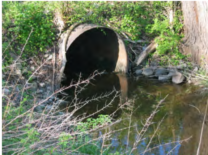
Picture #8 shows a 60" CMP crossing, under a private dirt path, on the Gilbert and West Town Intercounty Drain, near Station 30+00 in Section 24, Windsor Township, Eaton County.
