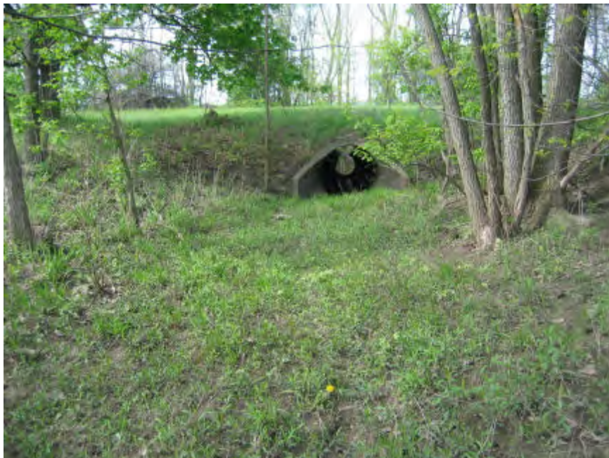
Picture #70 shows a 60" RCP and headwall on the south side crossing of the Gilbert and West Town Intercounty Drain under Interstate-96 west bound on ramp near Station 171+00 in the City of Lansing, Ingham County.
