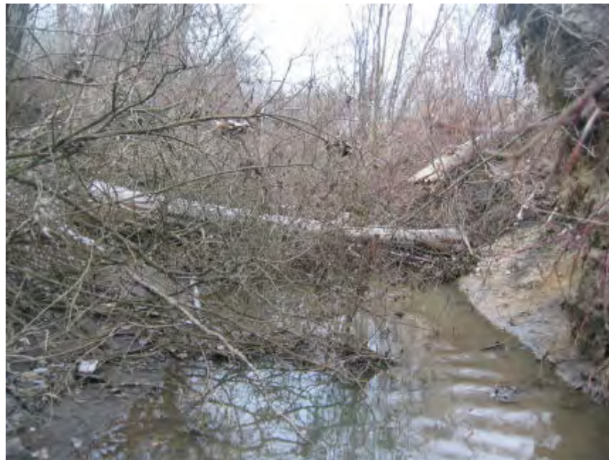
Picture #28 shows large fallen trees obstructing flow along the Gilbert and West Town Intercounty Drain near Station 81+00 in Section 18, Delhi Township, Ingham County.
