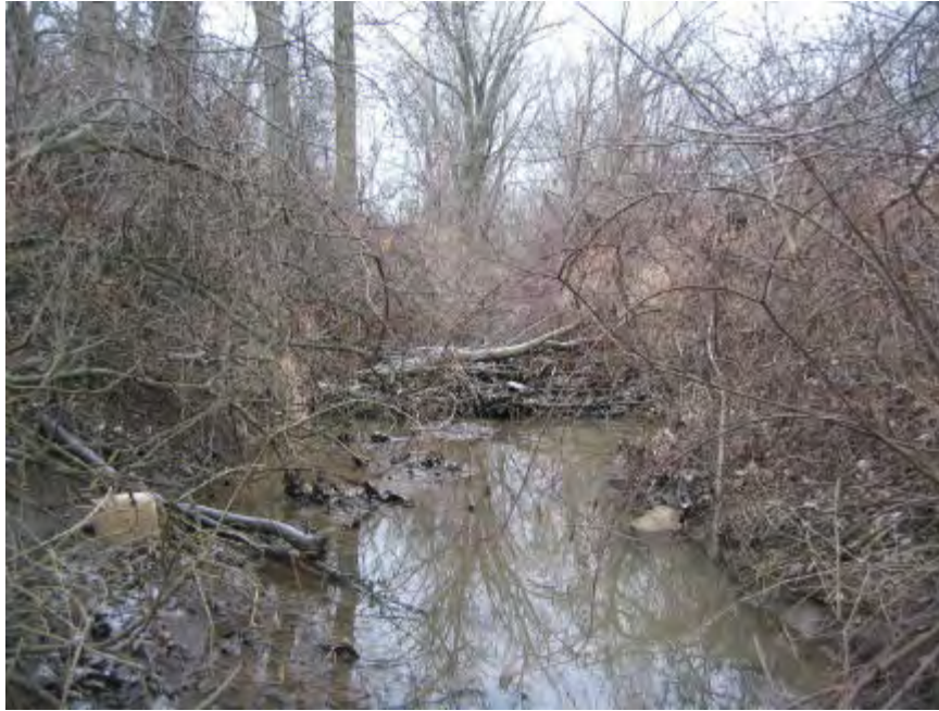
Picture #27 shows flow channel obstruction, logjams and debris buildup along the Gilbert and West Town Intercounty Drain near Station 77+00 in Section 18, Delhi Township, Ingham County.
