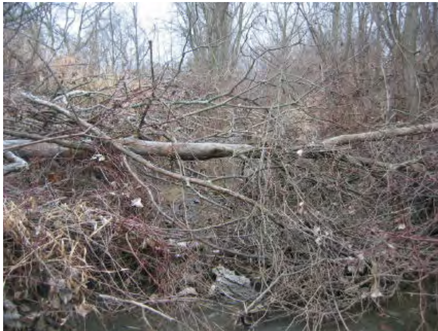
Picture #42 shows the Gilbert and West Town Intercounty Drain in with large fallen trees, logjams and flow obstructions near Station 122+00 in Section 18, Delhi Township, Ingham County.
