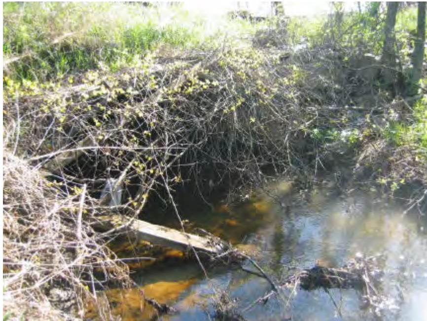
Picture #16 shows the Gilbert and West Town Intercounty Drain crossing on the south side of Holt Road near Station 59+50 in Section 19, Delhi Township, Eaton County. The crossing has a significant amount of overhanging brush and various flow obstructions.
