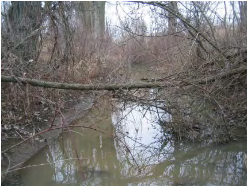
Picture #37 shows the Gilbert and West Town Intercounty Drain with fallen trees and debris build up near Station 109+00 in Section 18, Delhi Township, Ingham County.
