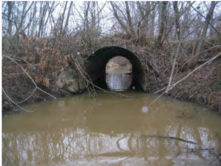
Picture #32 shows the south side of a 60" CMP crossing under a grass pathway on the Gilbert and West Town Intercounty Drain located near Station 96+50 in Section 18, Delhi Township, Ingham County.
