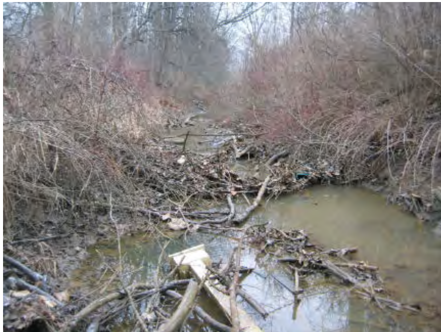
Picture #44 shows the Gilbert and West Town Intercounty Drain in poor condition with logjams, debris build up and heavy sediment build up near Station 126+00 in Section 7, Delhi Township, Ingham County.
