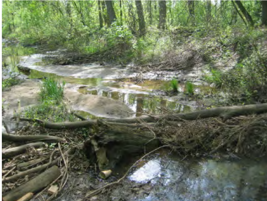
Picture #49 shows the Gilbert and West Town Intercounty Drain in poor condition with logjams, debris build up and heavy sediment build up near Station 134+00 in Section 7, Delhi Township, Ingham County.
