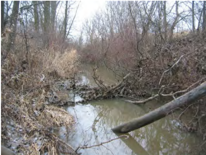
Picture #38 shows the Gilbert and West Town Intercounty Drain with flow obstructions and fallen trees near Station 110+00 in Section 18, Delhi Township, Ingham County.
