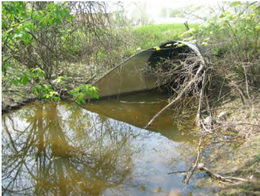
Picture #74 shows a 60" CMP of the Gilbert and West Town Intercounty Drain at its point of ending from its discharge point from the City of Lansing detention system near Station 182+50 in City of Lansing, Ingham County.
