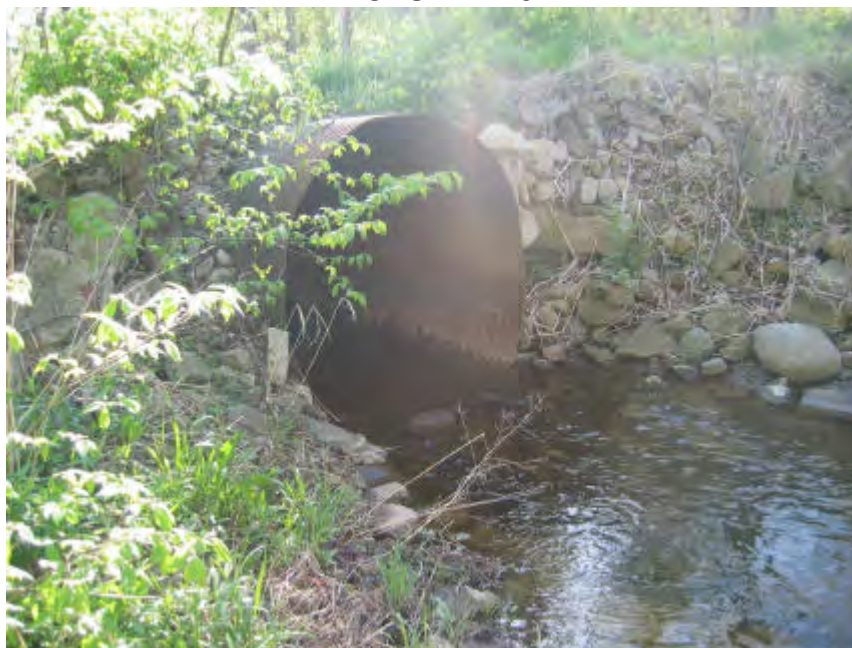
Picture #10 shows a 60" CMP crossing, under a private dirt path, on the Gilbert and West Town Intercounty Drain, near Station 37+00 in Section 24, Windsor Township, Eaton County.
