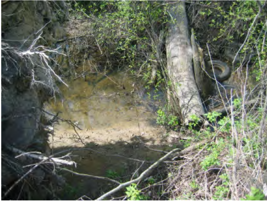
Picture #39 shows the Gilbert and West Town Intercounty Drain having eroded banks with logjams, debris and flow obstructions near Station 119+00 in Section 18, Delhi Township, Ingham County.
