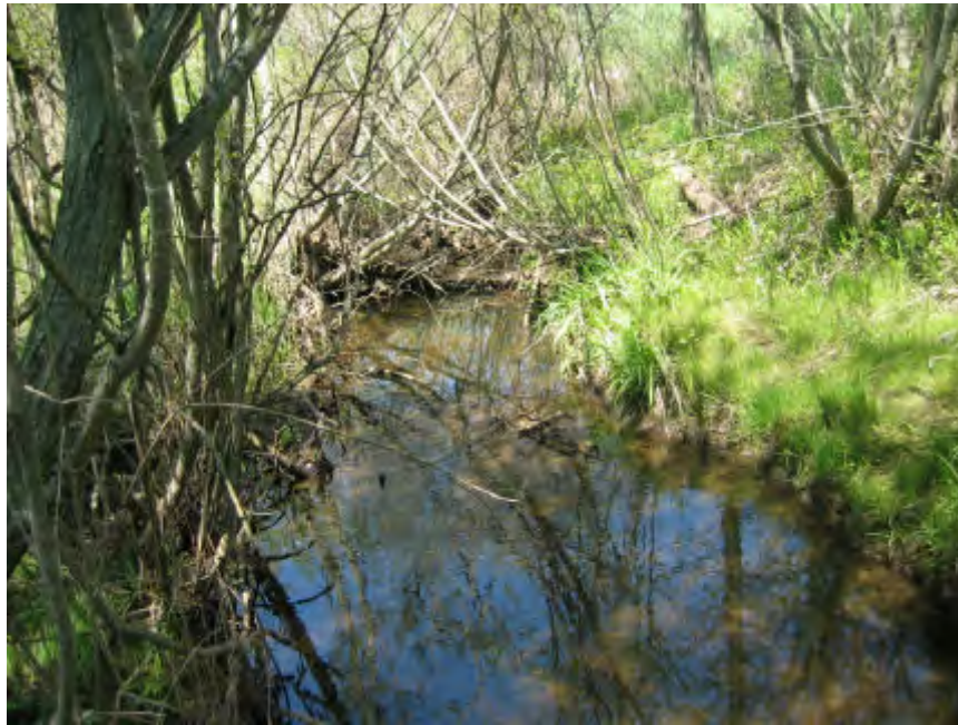
Picture #21 shows flow obstructions, overgrown brush and logjams along the Gilbert and West Town Intercounty Drain looking north located near Station 67+50 in Section 18, Delhi Township, Ingham County.
